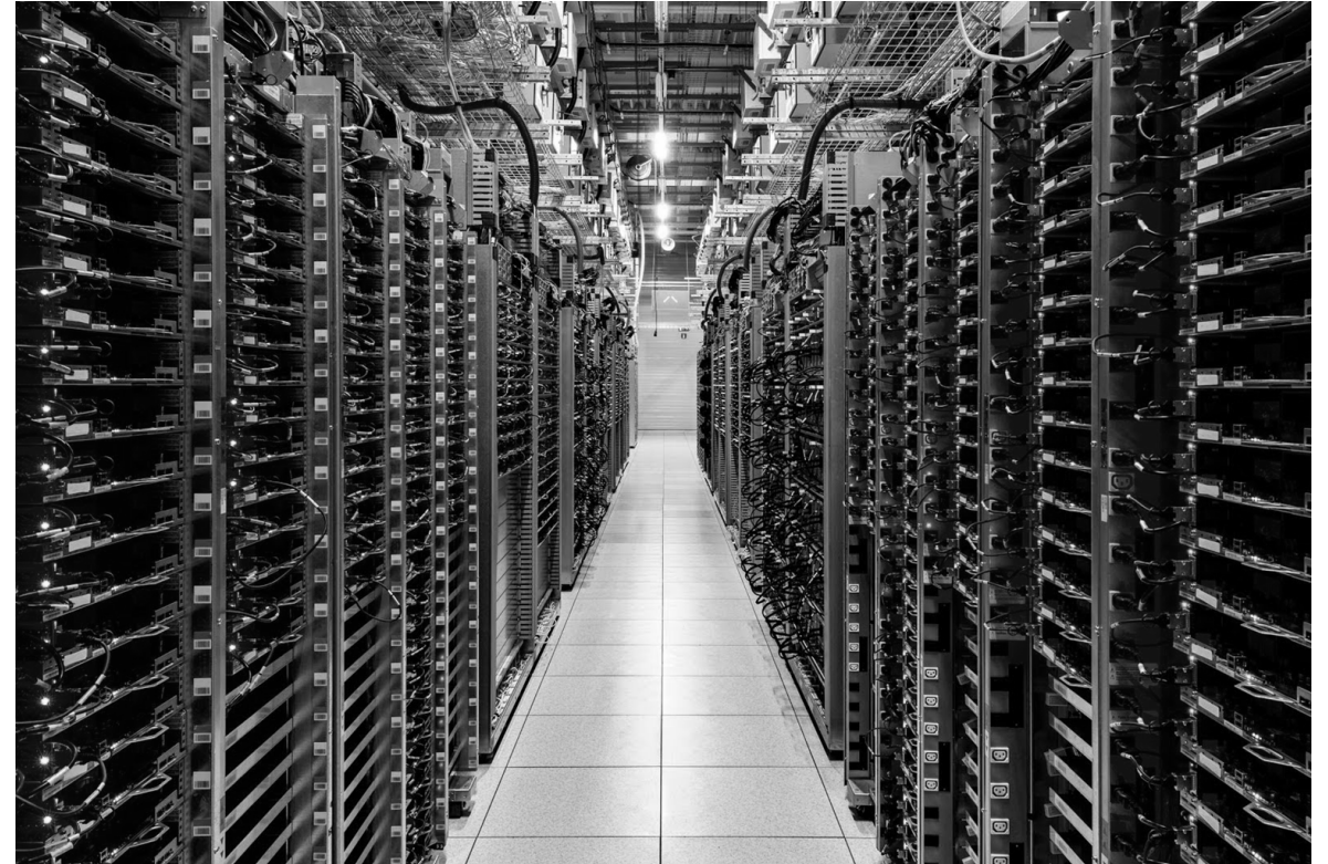
Servers light up in our St. Ghislain, Belgium data center. (Google Data Centers Photo Gallery)
