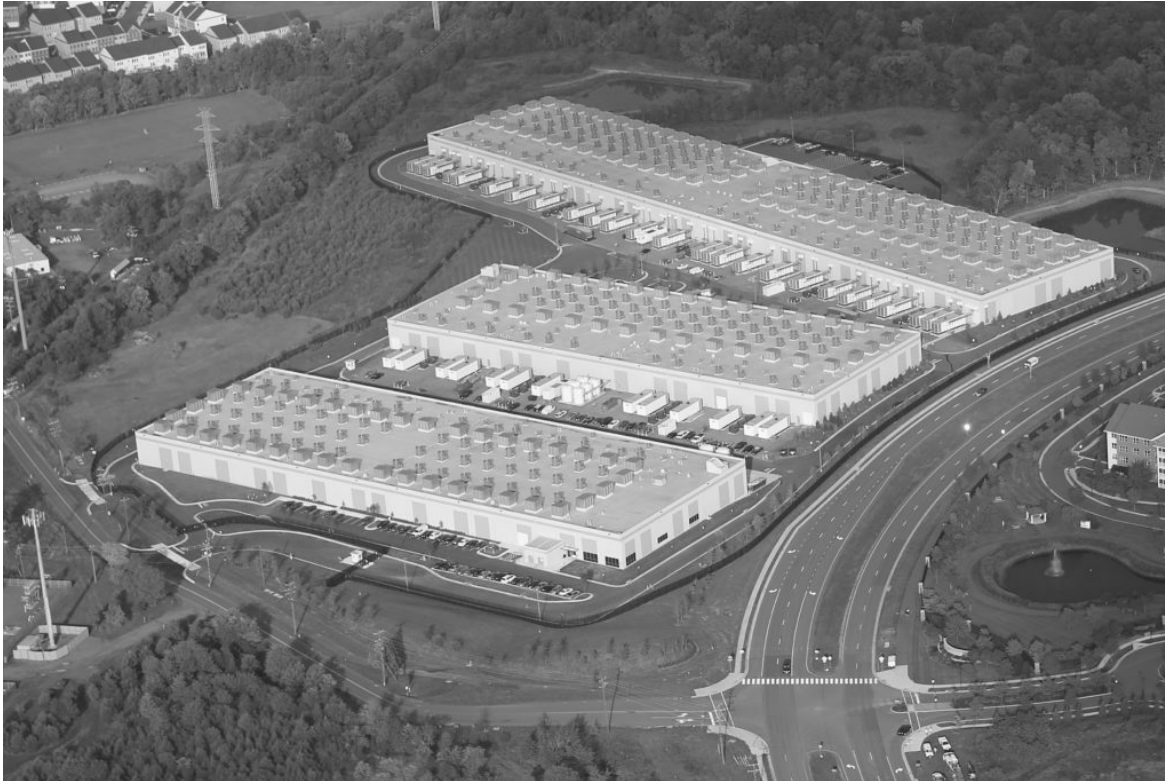
An aerial photograph of one of Amazon's data centers near Dulles International Airport in northern Virginia. (Carolina Journal photo by Don Carrington)
